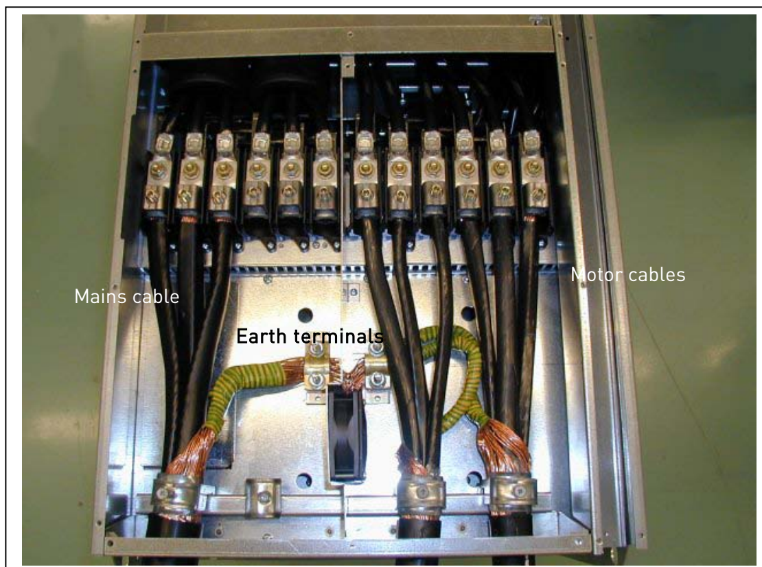
Figure 6-22. Cable installation in Vacon NXS/P, FR9
