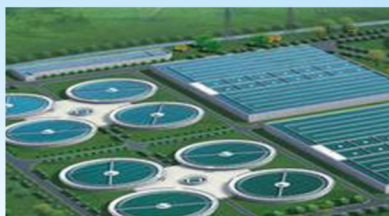
Sewage treatment plants
